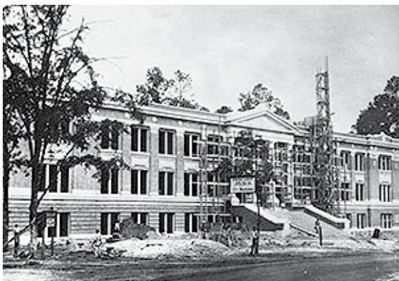
The Rusk Building under construction in 1926.
