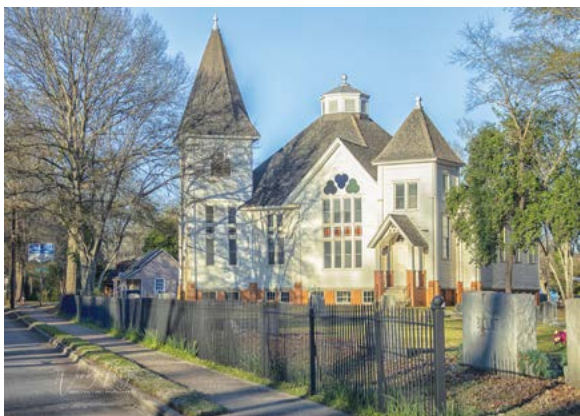
Zion Hill Baptist Church, completed in 1914 and recently remodeled, was designed in a Gothic Revival style by Diedrich Rulfs.
